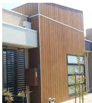
4 MONTHS: The board shows signs of lightening.
